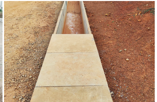
Laying Cover Slab
